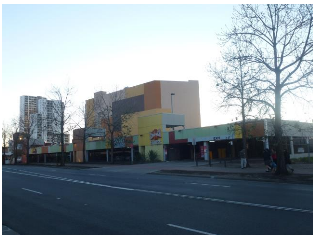
Figure 6: Above ground car parking structure as viewed from Terminus Street (south east)
