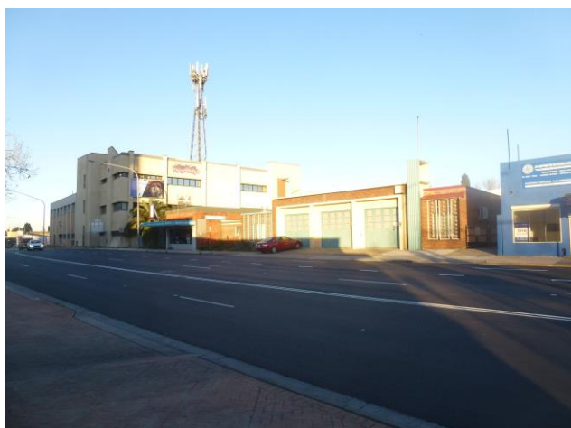
Figure 17: Telstra Exchange building and adjoining retail tenancies to the south
