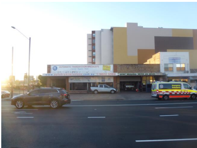
Figure 21: Rear party wall presented to the site
